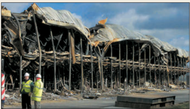
Half of the Yarl's Wood Detention Centre in Bedfordshire, England, was destroyed by a series of fires Feb. 14-15.
