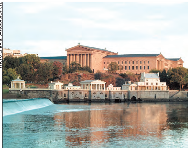
The Fairmount Water Works, shown here with the Philadelphia Museum of Art in the background, was built in 1815 and once pumped 4 million gallons of water daily from the Schuylkill River to a reservoir.
