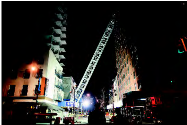
Part of a large crane collapsed in Midtown Manhattan last month, killing seven people. Less than two weeks later, a crane accident in Miami killed two others.
