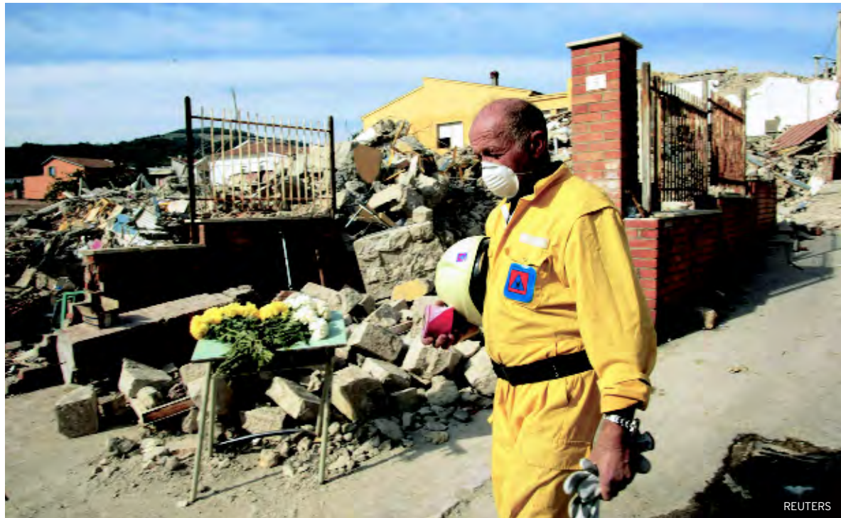
A school in San Giuliano di Puglia, Italy, about 140 miles from Rome, collapsed in 2002 after an earthquake and killed more than two dozen people, most of them students at the school.
