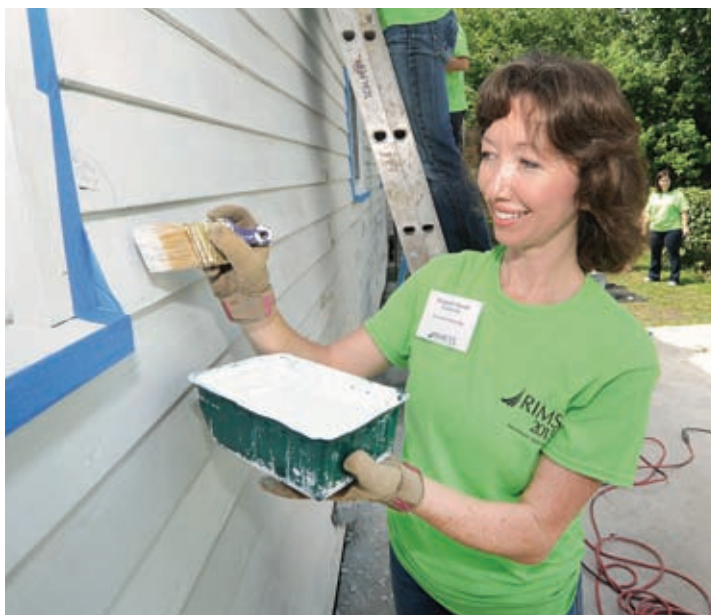
Elizabeth Morrell, principal, Silvient Inc., was one of many volunteers working to rebuild homes destroyed by Hurricane Katrina.
