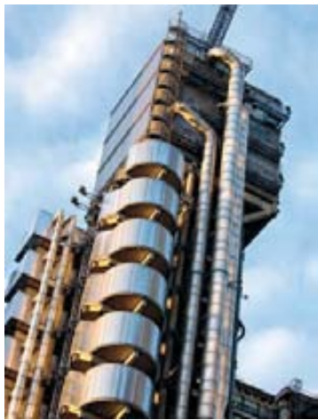
Lloyd's this year introduced a risk code for cyber security property damage.
