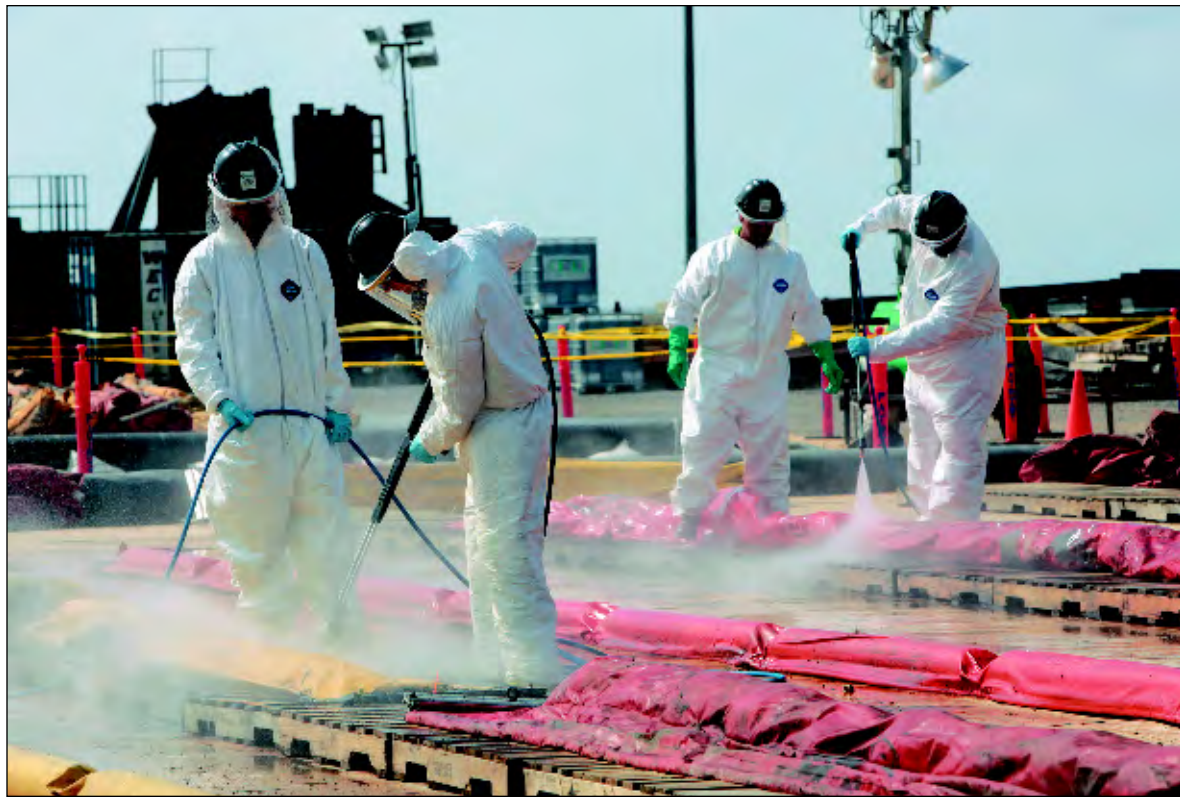
Oil cleanup workers use high-pressure hoses to decontaminate retention booms used to contain oil from the Deepwater Horizon spill in the Gulf of Mexico. BP P.L.C. and its contractors will face an array of injury claims, experts say.
