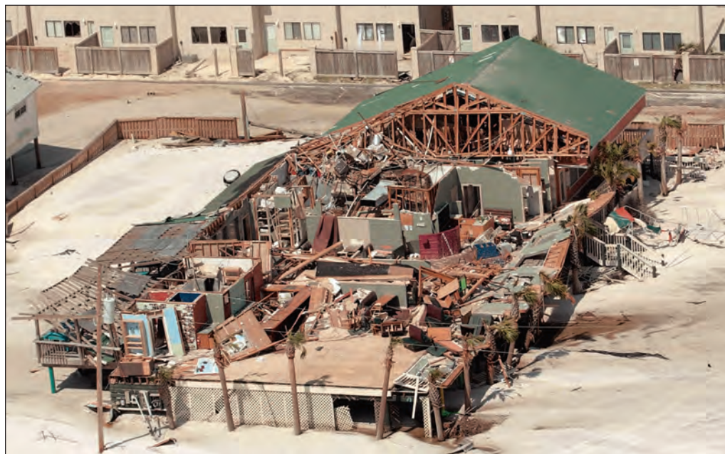
Some businesses in Navarre Beach, Fla., were flattened by Hurricane Dennis, but total insured damage from the season's first hurricane to make landfall was lower than expected.
