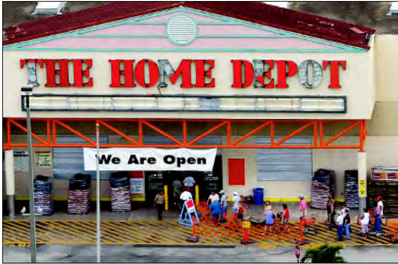
Despite damage to its facility, a Home Depot in Stuart, Fla., was open in early September 2004 for those seeking materials following Hurricane Frances. ZUMA PRESS
