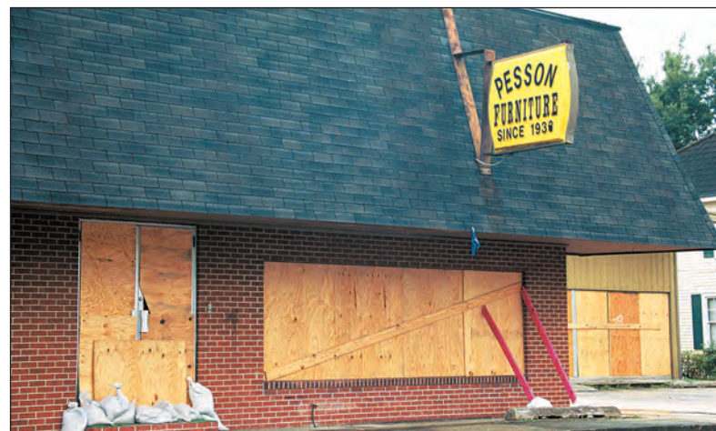
Plywood and sandbags can help mitigate the possible damage from hurricane-driven rain.
