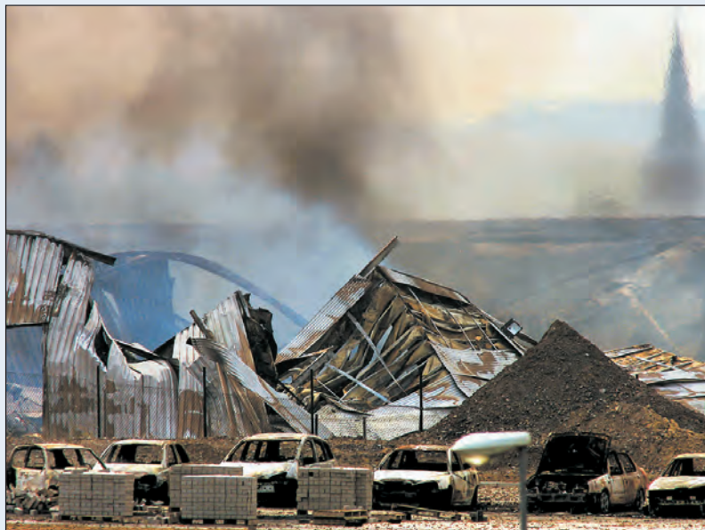
A blast at a natural gas pipeline late last month killed 17 and damaged buildings in an industrial park in Ghislenghien, Belgium.
