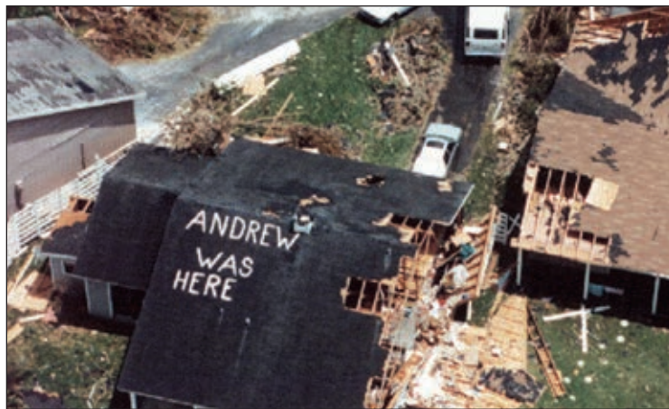
Hurricane Andrew caused widespread damage in Florida in 1992. After the storm, insurers changed their approach to catastrophe underwriting.
