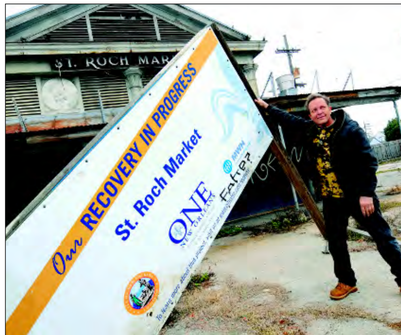
St. Roch Tavern owner John Victorson props up a reconstruction sign in February. New Orleans' St. Roch Market has yet to be rebuilt since Hurricane Katrina.
