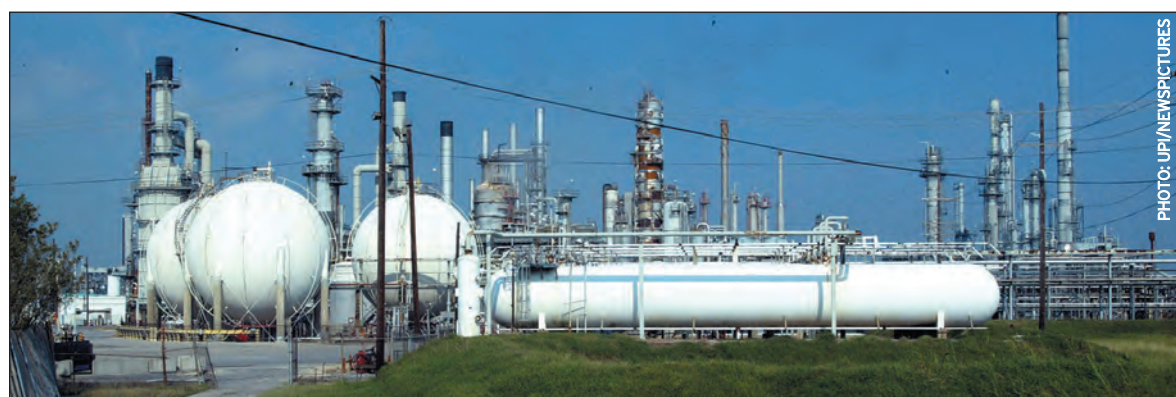
Murphy Oil USA Inc.'s oil refinery in Meraux, La., comes back on line after Hurricane Katrina.
