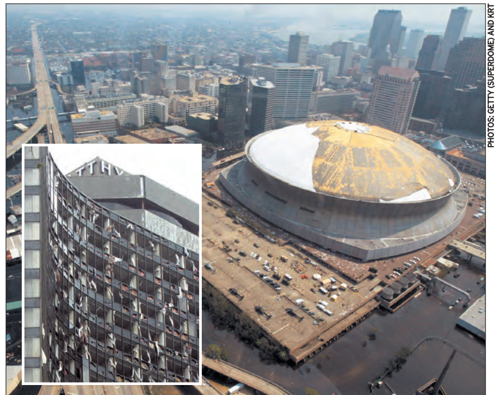
The Superdome in New Orleans, which served as a shelter for thousands of city residents during the hurricane, sustained damage from the storm's winds and rain. The facade of the Hyatt Regency, inset, in the city also was heavily damaged by Katrina.
