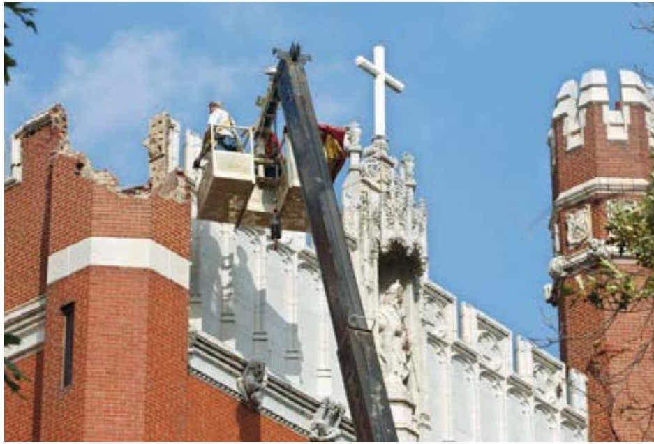
Maintenance workers inspect a spire on Benedictine Hall at St. Gregory’s University in Shawnee, Okla., which toppled after two earthquakes hit in less than 24 hours in 2011.
