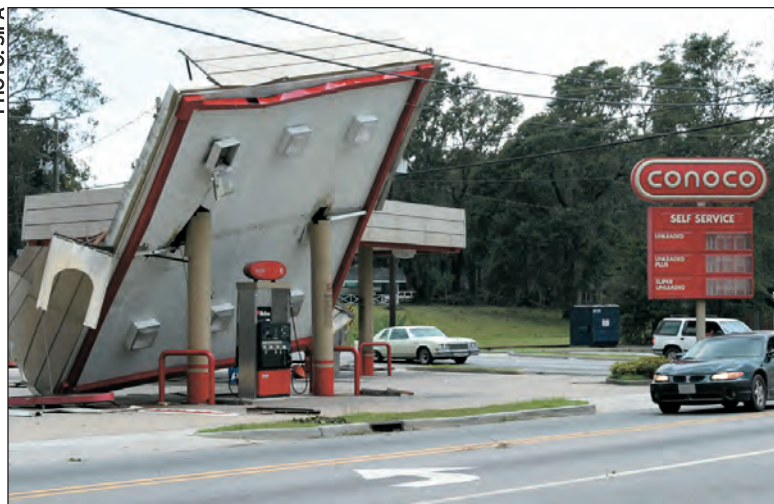
Properties in Mobile, Ala., such as this gas station, were severely damaged when Hurricane Ivan pounded the state last month.
