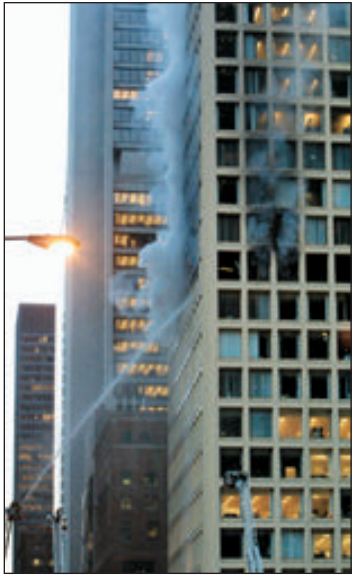
Firemen try to control a blaze at the Cook County Building in downtown Chicago. Officials have not determined the extent of the loss.
