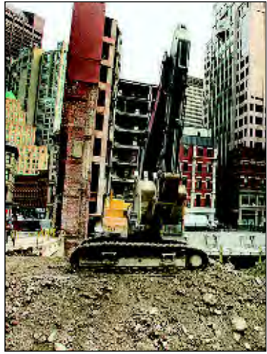
Construction at a site in Boston was halted in August because the main investor allegedly ran out of funding.
