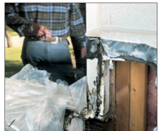
An inspection of a house in McKinney, Texas, uncovers mold and damaged lumber framing behind plastic foam.
