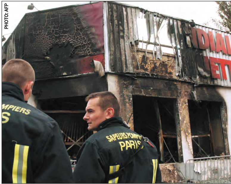
Firefighters in Bondy, France, inspect a riot-damaged carpet store.
