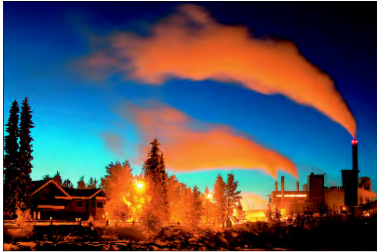
Steam rises from the Aurora Energy plant in Fairbanks, Alaska, in 2005. The plant supplies Fairbanks with power.
